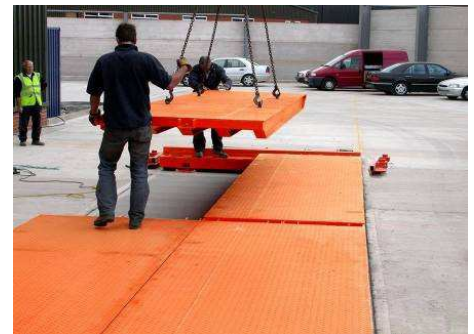
Simple drop in place sections
